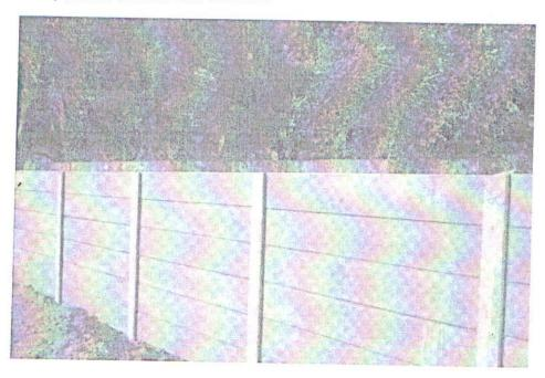
2 RCC Precast Pre-Stressed Plank (2100mm X 300mm X 50mm Plank with 4 bars of 3mm HTS Steel with M-30 Grade Of Concrete Used
