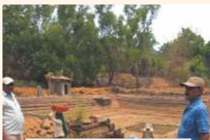
Rejuvenation under progress
