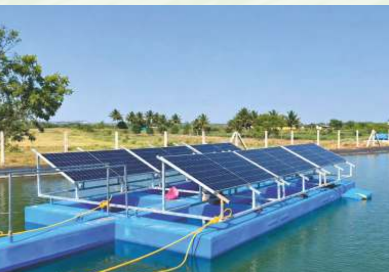
Floating Solar Panel on farm ponds for energy generation
