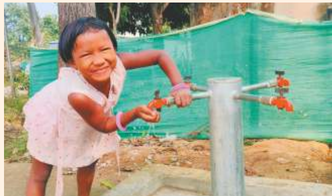
Clean drinking water system for improved health
